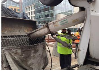
Concrete is delivered to pumps on the Transbay site for the project's mat slab, walls, columns and other concrete elements
