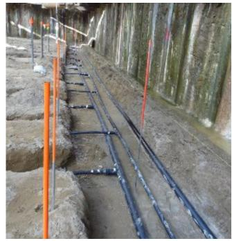
Geothermal piping under the foundation of the Transit Center will reduce heating and cooling needs for the Transit Center, helping to achieve a LEED Gold rating.
