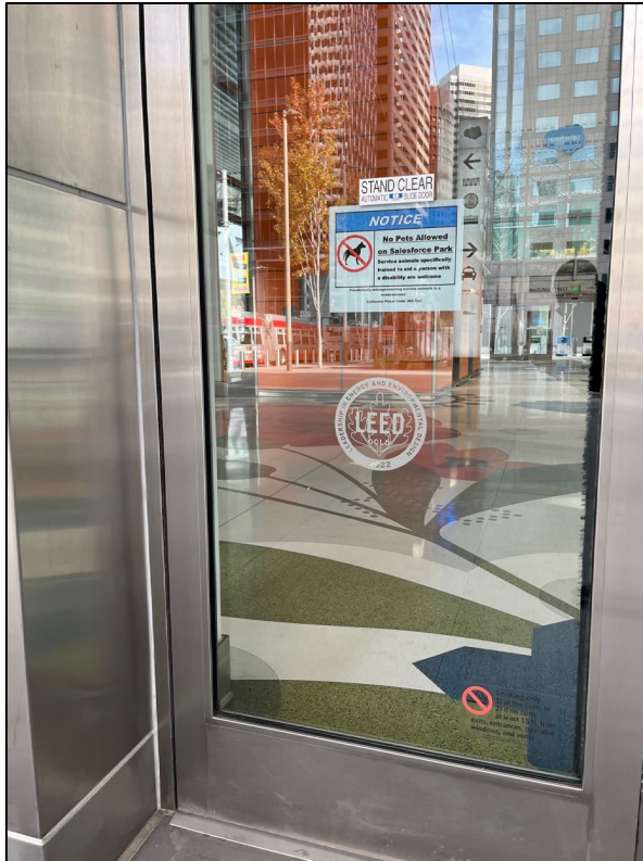
LEED Gold Decals Installed.
